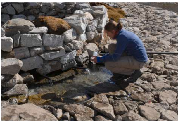
Fig. 3. Drinking water source in Lobuche. A stone wall fence prevents livestock from accessing the water source directly, but they may drink below the outflow. Tubes facilitate the filling of containers. (Photo: T. Küpper).
